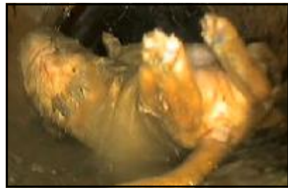
"Dyno" being gently pushed along pipe.
